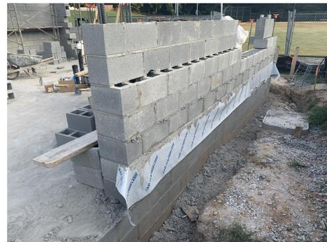
FD- Block wall transition in preparation for architectural transition detail
