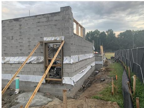
FD- Block out installation for future glass block, louver, and roll up doors
